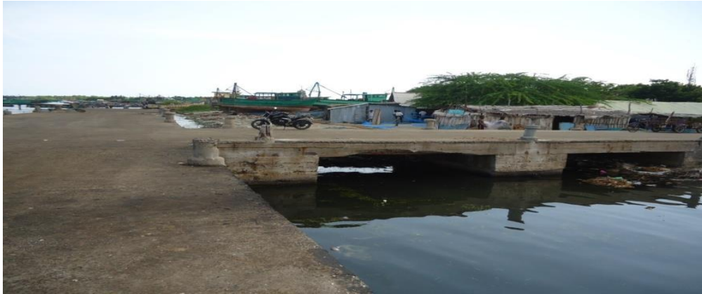
Picture 6.1: The Status of Fish Basin in Rameshwaram Jetty
